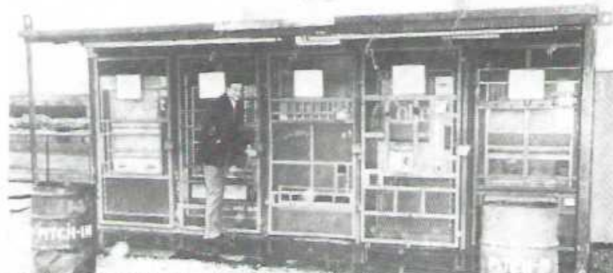
MODULAR BANK: Alan Kronenberg of Food Management Corp. checks one of the firm's self-contained outdoor vending kiosks on the grounds of Avondale Shipyards (Metairie, LA). Durably constructed and equipped with lifting-bits (visible at top left and right), the kiosks can be lifted by huge shipyard cranes and set down on concrete foundations pre-installed at various places in the shipyard. As new vessels are laid down, kiosks are moved into the work area to serve the builders.
